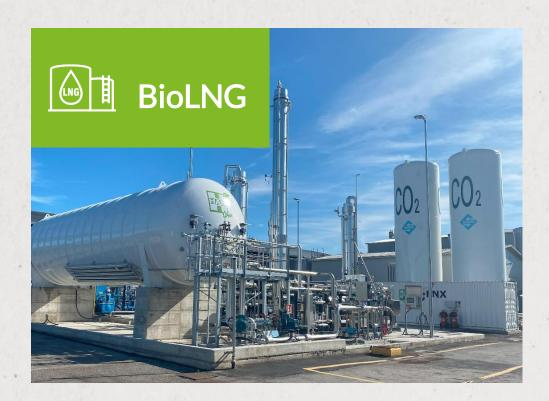
Biomethane, produced by agri-food industry waste, is brought to liquid form in order to optimize its use in the heavy vehicle sector.
