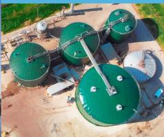
The Extra Eco-Energy division is located downstream of the recycling cycle and transforms waste, effluent and digestates into energy and soil improvers for agriculture.
