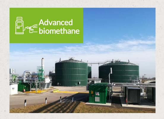
Thanks to the anaerobic digestion of agri-food industry waste, every year
